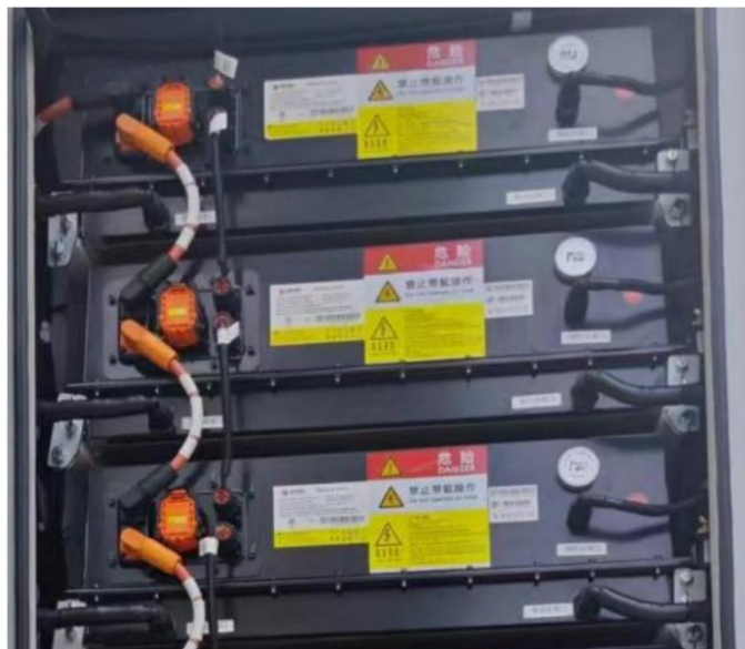
Figure 6-6 Adjacent battery packs after connecting the high-voltage cables and communication cables
