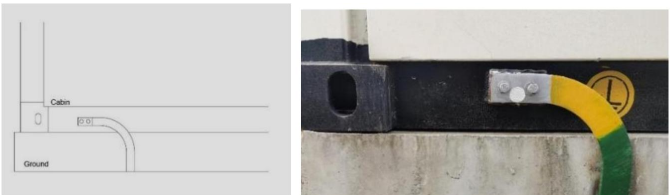
Figure 5- 12 On-site grounding of the ESS container
